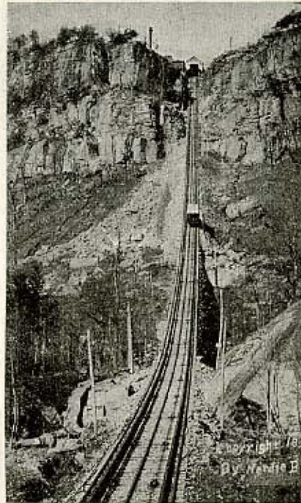
PARTIAL VIEW OF THE INCLINE UP LOOKOUT MOUNTAIN, CHATTANOOGA.
